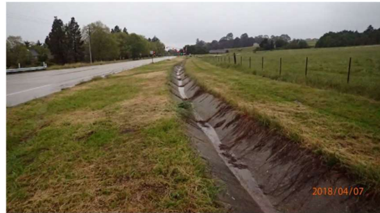
V-channel along Coolidge after rain has cleared debris
